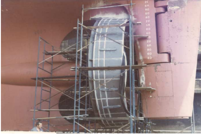
Figure 5.4 Cracks in slotted nozzle of 'John Ross' after trials
